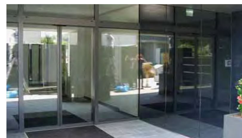
Entrance to the premises of Hilti AG
